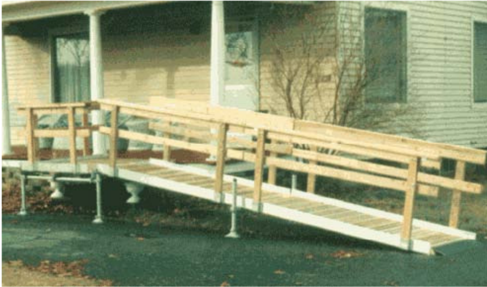
A modular L-shape ramp
